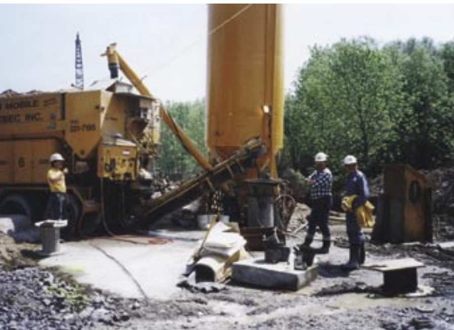
Fig. 4: Stationary concrete mobile mixer supplying wet-mix shotcrete for effluent outfall tunnel, Bécancour, QC
