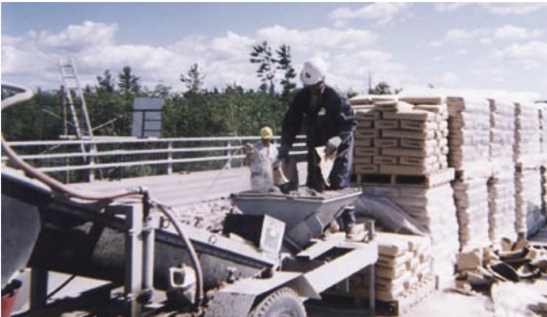
Fig. 2: Dry-mix prebagged shotcrete used with predampener for repairs to Hydro-Québec Dam in Fort Coulonges, QC
