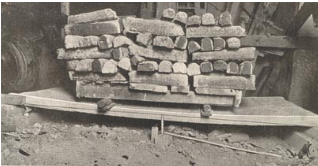
Test of gunite slabs made under supervision of Professor M.O. Fuller, Lehigh University. (The tests were started in 1920 and ran through 1934. The 8 ft [2.4 m] span, 3-1/4 in. [82.6 mm] thick, deflected 2 in. [50 mm] by 1922 and stressed the reinforcing to 36,000 lb [160 kN] at completion. No further deflection occurred after the 3rd year.)
