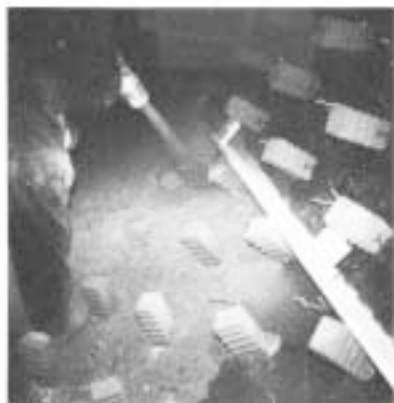
Fig. 20: Ceramic anchors interspersed with corrugated V-Clips.
