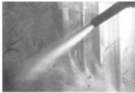
Fig. 17: Bench gunning or 45 deg angle nozzle technique.
