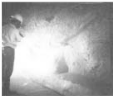
Fig. 17: Bench gunning or 45 deg angle nozzle technique.
