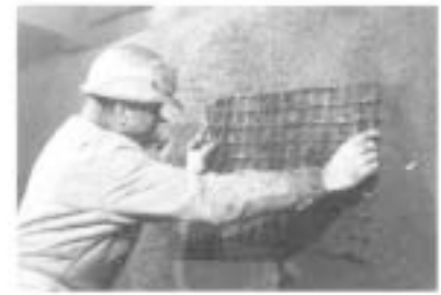
Fig. 18: Removing high spots after gunning.
