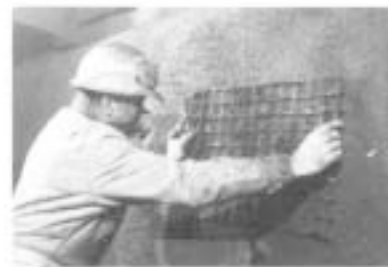
Fig. 18: Removing high spots after gunning.
