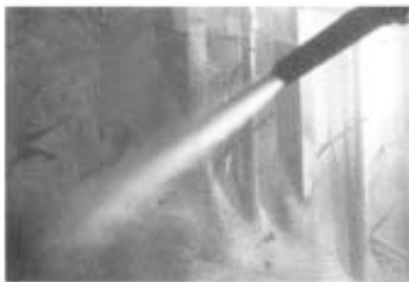
Fig. 17: Bench gunning or 45 deg angle nozzle technique.
