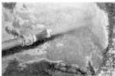
Figure 23: Hot gunning a ladle, lower area about 1500 to 1700° F (816 to 927° C).
