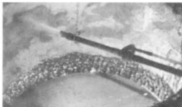
Figure 22: Hot gunning refractory shotcrete lower area is red-orange heat.
