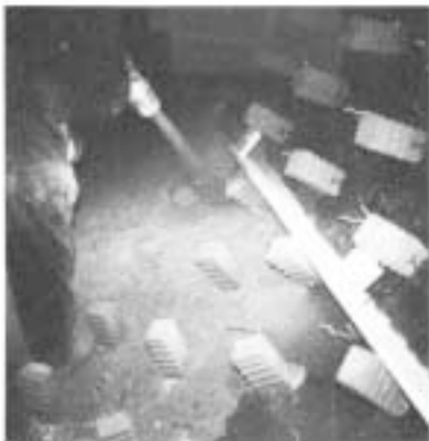
Fig. 20: Ceramic anchors interspersed with corrugated V-Clips.
