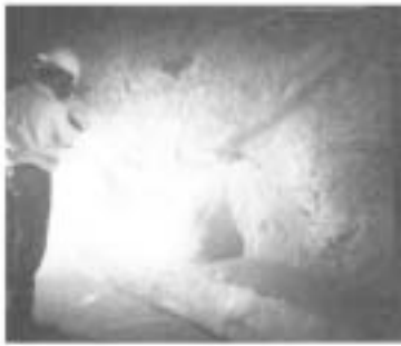
Fig. 17: Bench gunning or 45 deg angle nozzle technique.
