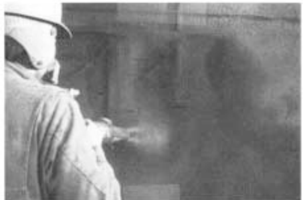
Figure 16: Right angle nozzle technique.
