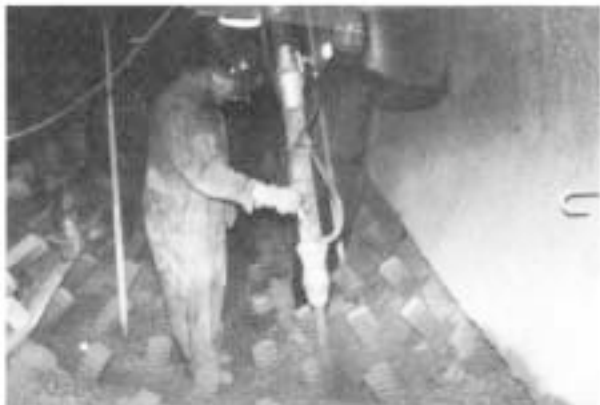
Figure 15: Gun casting (note completed section at upper right).
